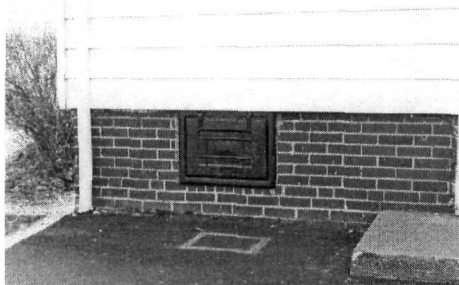
Coal chute, 1101 Droukas Court, view south (photo by James Jacobsen, December 7, 1999)
