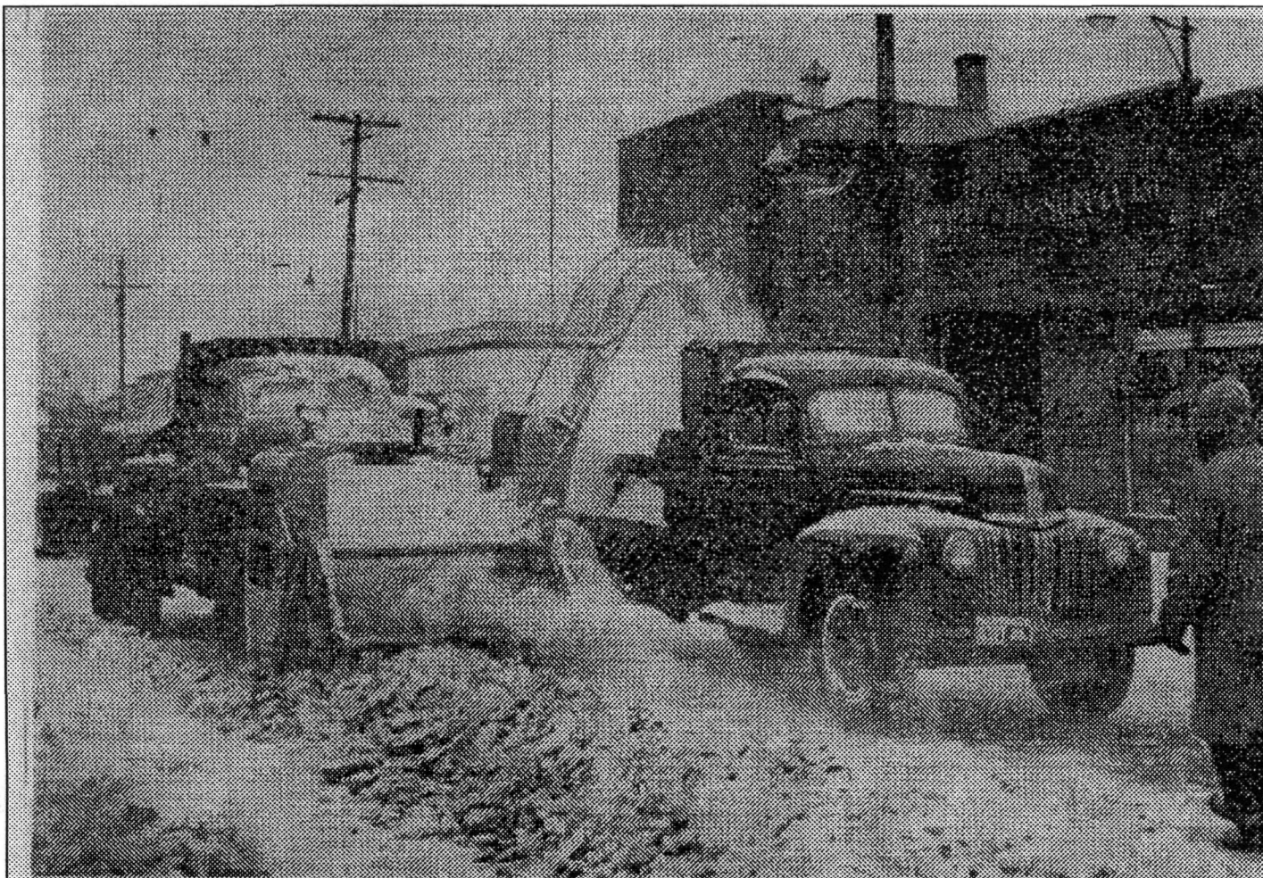
Among the equipment being used to remove snow from Des Moines streets this week is rotary type plow built by a Cedar Rapids firm and being demonstrated "on the job" by a factory representative. Here it is cutting away packed snow along Sixth avenue in Highland Park.
